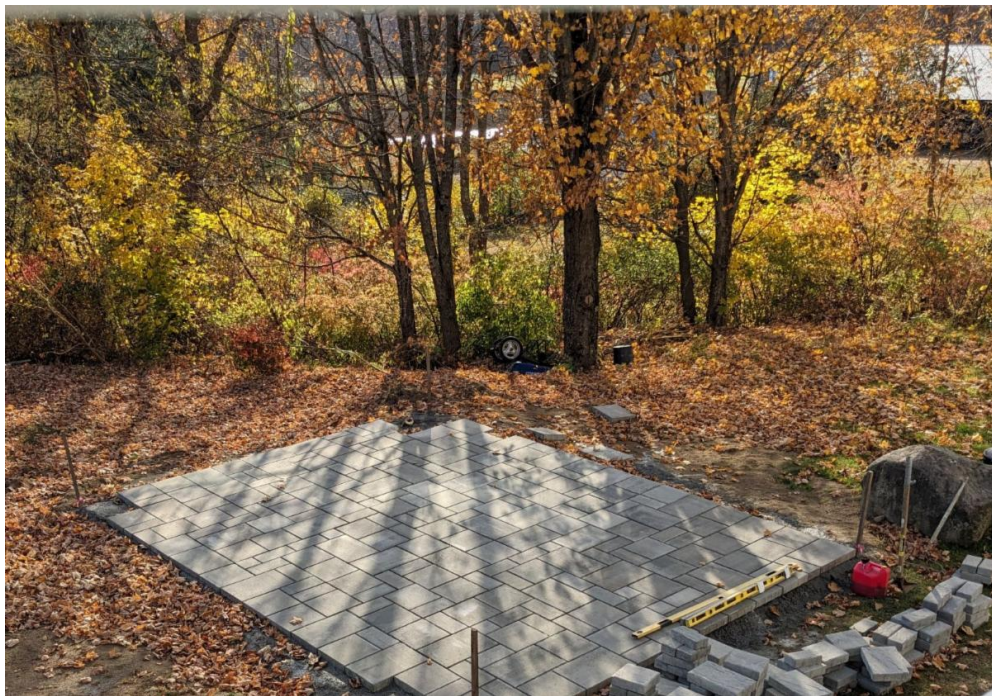
Gazebo foundation takes shape....
